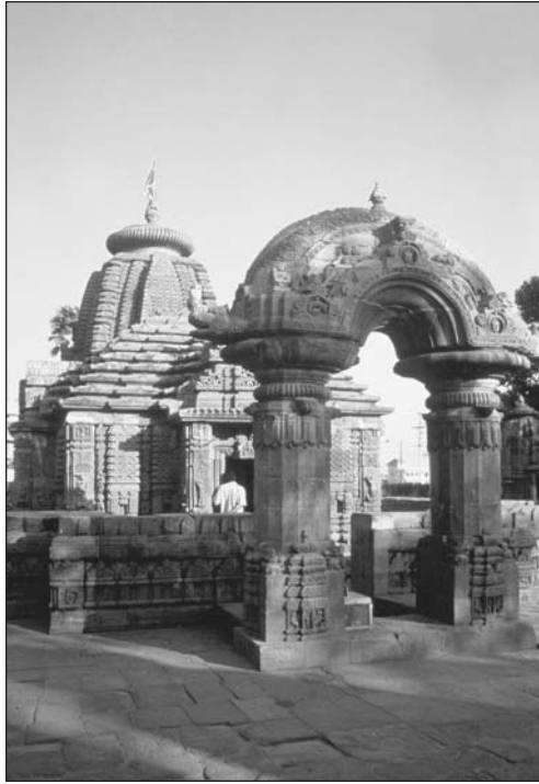
The architectural technique of corbelling was used to form the arched entrance to the Mukteshwar Temple in Bhubaneswar.
